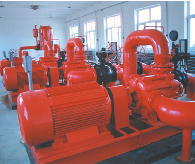
连成XBD-D卧式多级消防泵组有效地运行在工业企业的消防系统。 Liancheng XBD-D Horizontal Multi-stage Fire Pump Unit works effectively in the fire-fighting systems of industrial enterprises.
